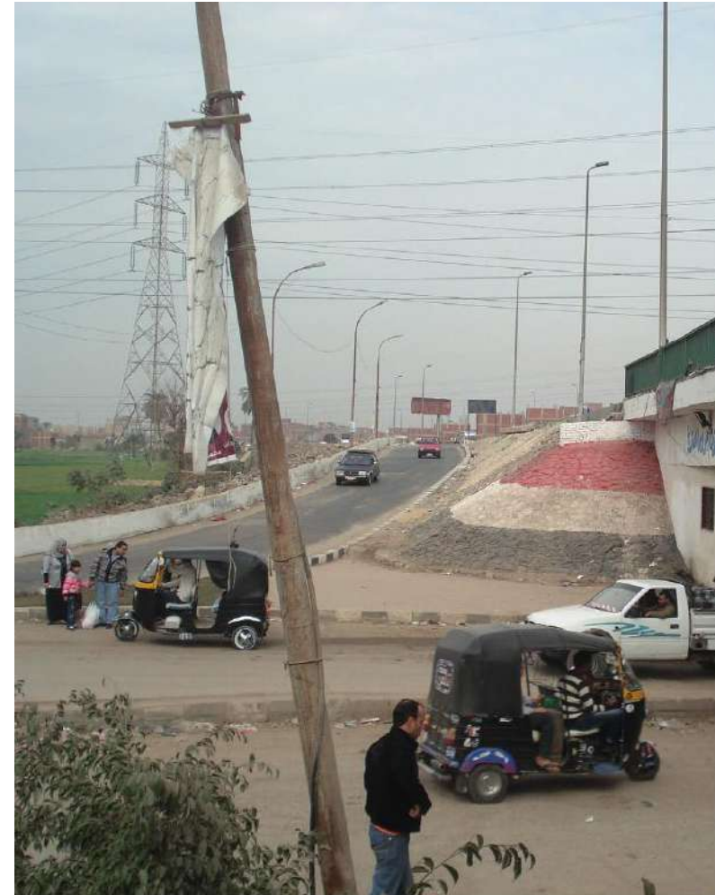
Figure 17. - The Al-mu'tamidiya exit, an informal ramp constructed by a grassroots community initiative allowing vehicular access onto Cairo's ring road.
