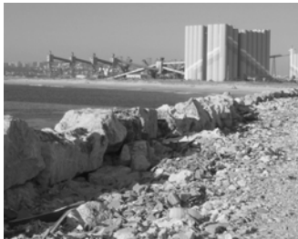
Riprap protects coastline against erosion
